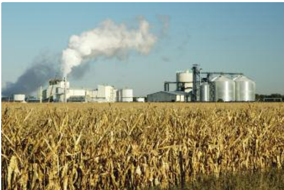
A fuel ethanol plant in the US mid west.
